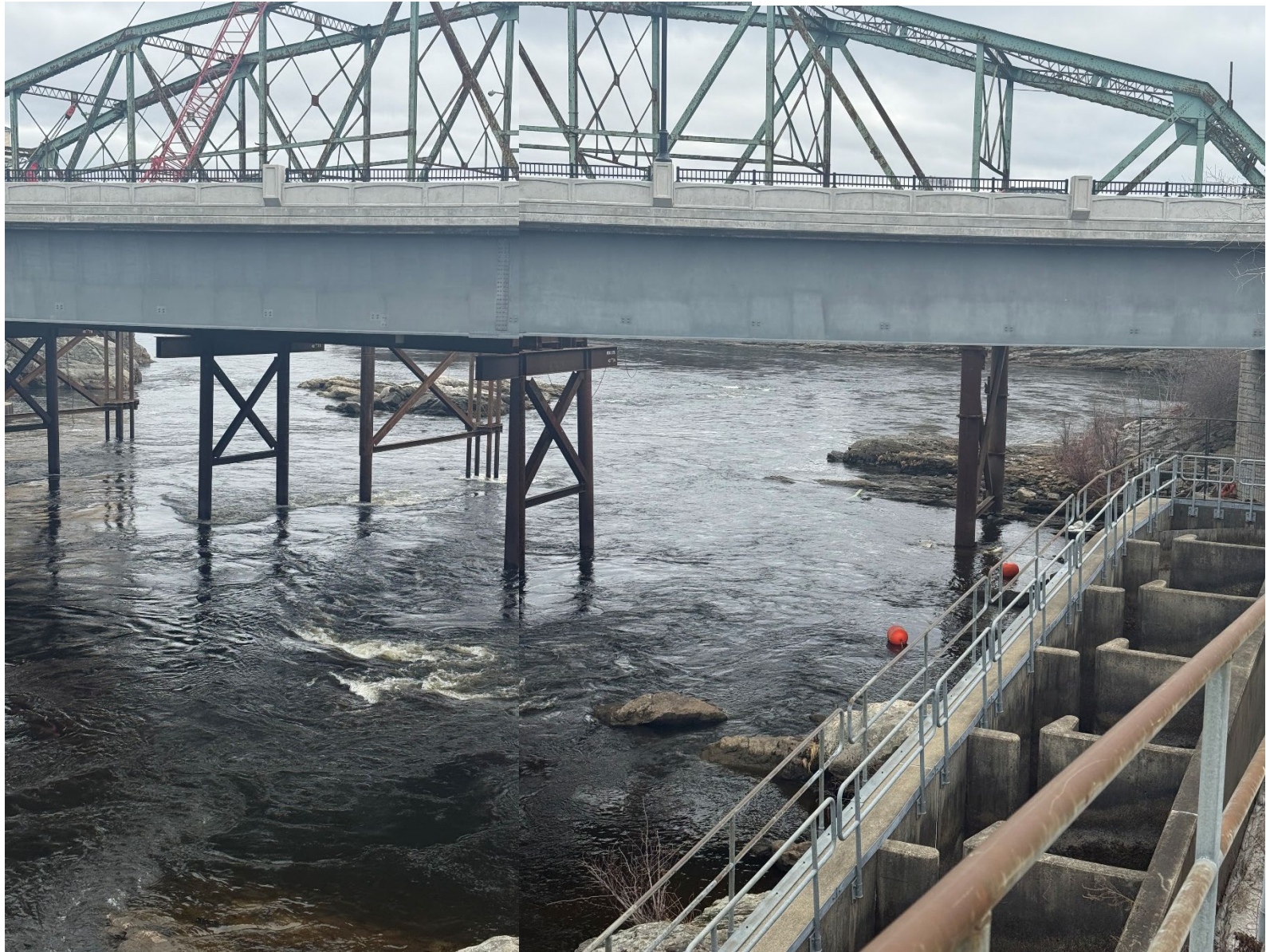
Figure 2: Photograph of Steel Piles Supporting the Work Trestle and Old Bridge
